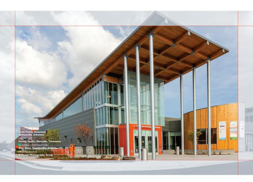
It's hard to say whether the beauty of the 1620/1620 SSG (structural silicone glazed) Curtain Wall System is in the slim, sleek 2" sightline or in the performance. Built on the strength and reliability of the flagship 1600 curtain wall platform, the 1620/1620 SSG Curtain Wall System is an excellent choice for low- to mid-rise applications.
